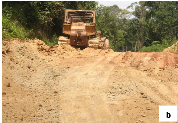
Figure 3. Heavily degraded area; (a) timber transport road, (b) a caterpillar machine in the process of constructing timber-transport road.
