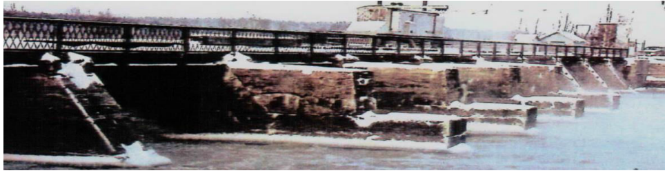
Figure 2. Illustrating the Dam site and its harsh Environmental Conditions.
