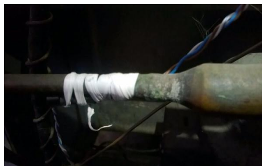
Fig.III.VIII Condenser temperature sensor
