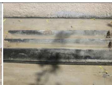
Fig (7) (a): Curing of panels
