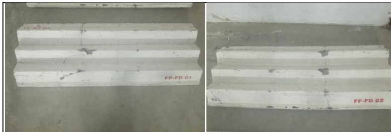
Fig (12) (a): Crack pattern FP-FD 01 Fig (12) (b): Crack pattern FP-FD 02
