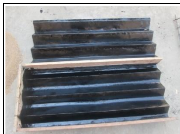
Fig (4): Fabrication of mould
