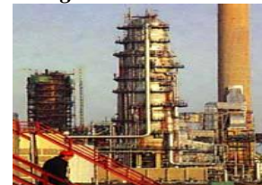
Figure 10: A Distillation Tower
