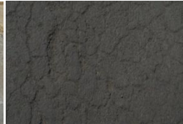
Fig.6 Map Cracking
