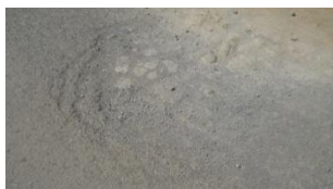
Fig.3 Map cracking
