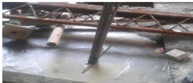
Figure 3: Grouting
