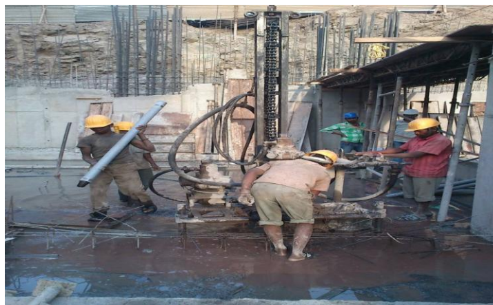
Figure 2: Drilling of Bore Hole
