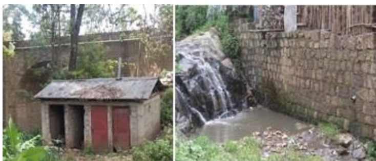
Fig. 1. Public and residential toilets directly opened to Walgamo river.
